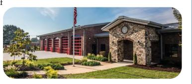
trusses, and for the bays a pre-engineered metal building. The roofing material is standing seam metal roof that will withstand the elements for many seasons.
